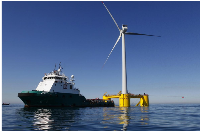
Figure 1: Maneuver of installation of the Windfloat device towed by a PSV.
