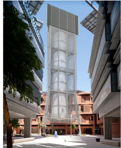
A modern interpretation of the Arabian wind tower is used to cool the plaza areas at the Masdar Institute of Science and Technology
