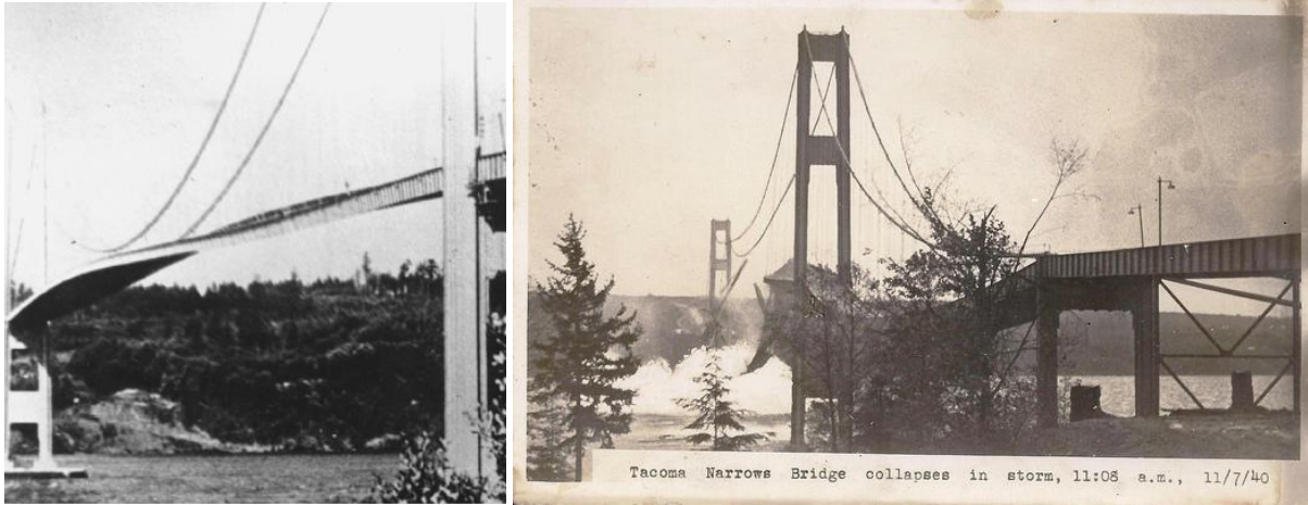
Figure 3 Tacoma Narrows bridge failure incident
